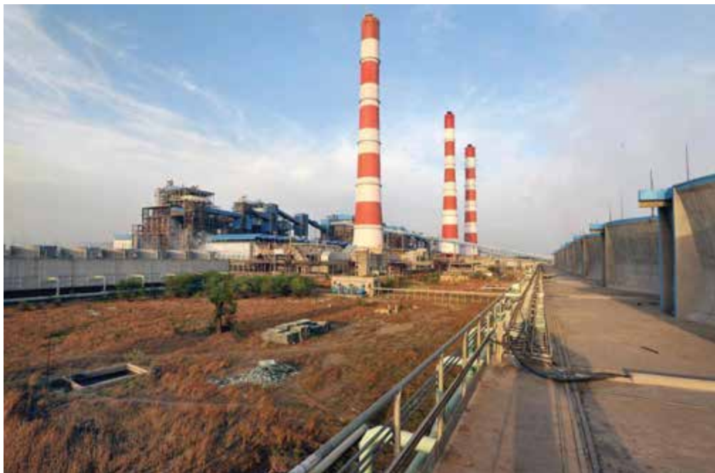
National Thermal Power Corporation Barh STPP located in Barh, Patana district, India.
