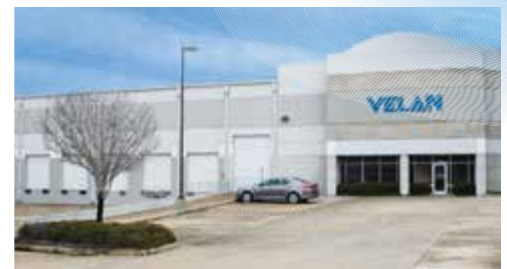
Outside view of the new VelTEX distribution center.
